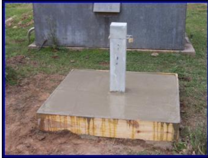
Figure 7A-2 Example of outer protective steel casing with a hinged, locking cap
